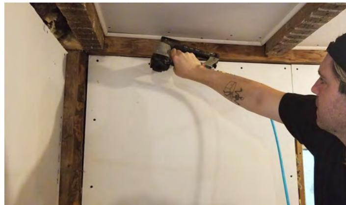
Ben Fama uses a nail gun to install quarter round trim around the ceiling drywall.
