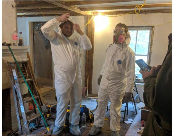
Proper precautions were taken before scraping the old lead paint.
