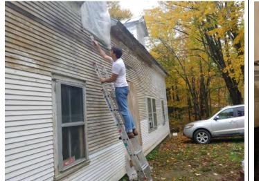
Ted Dodson applies wood filler to holes purposefully bore into the house to install installation sometime mid 20th century.
