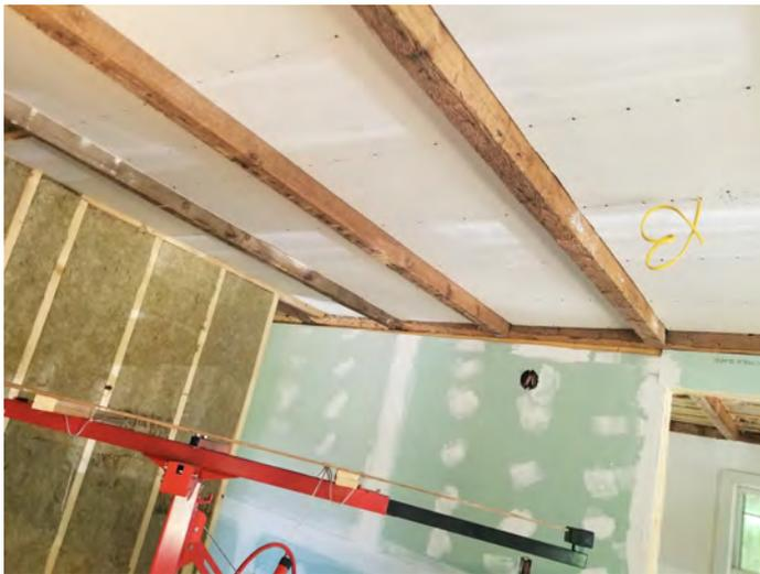
One wave of drywall installed with a hoist lent to the foundation by neighbor Brian Ford.
