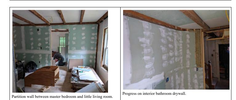
? hours + \$15 for a bucket of joint compound (No one likes taping drywall, so Ben finds himself doing it in between other jobs, losing track of time as he scraps the combination of gypsum dust and water over screws and joints to make many pieces appear as one).
