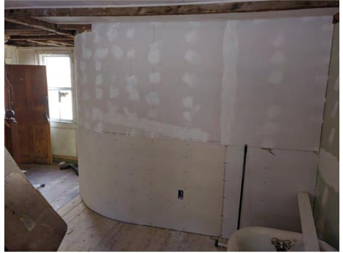
Curved pieces installed onto bathroom wall and partially taped.
