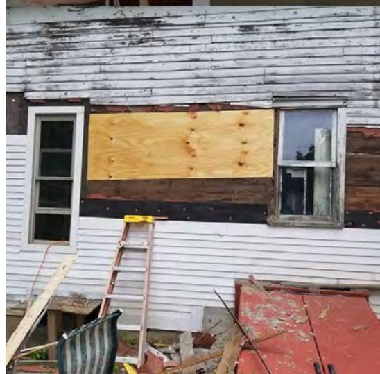
Clapboards to the left of the leftmost window approach its top while installation had to wait in between the two windows until the sheathing could be replaced.
