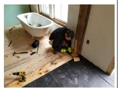
After using a small block and wedge to get the often curved floorboards straight against the previous one, the Guy Pettit uses a combination square to mark and pre-drill holes for the nails.
