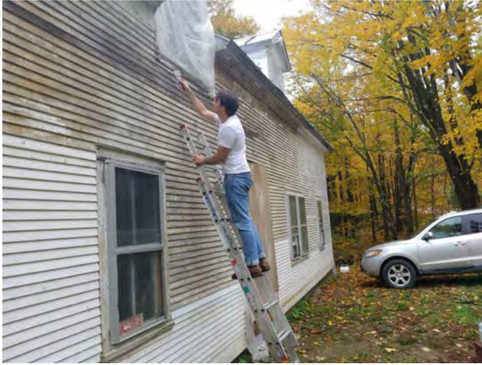
Ted Dodson applies wood filler to holes purposefully bore into the house to install installation sometime mid 20th century.
