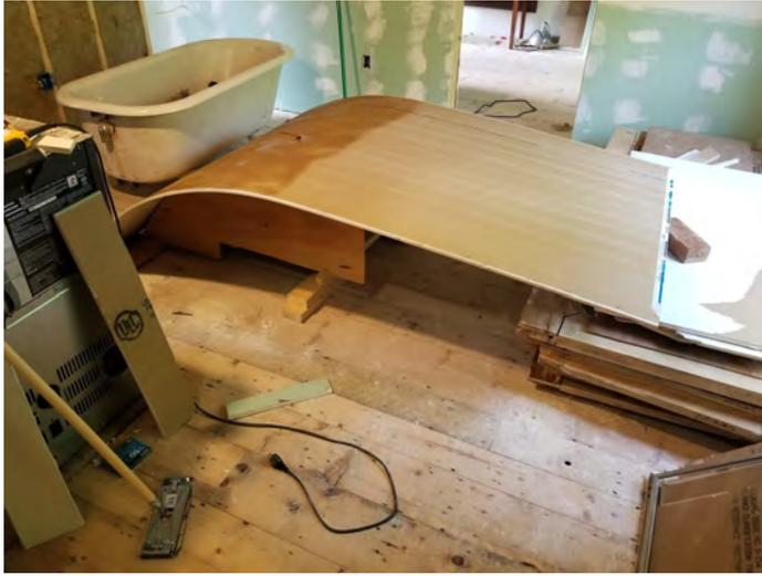
Custom-made frame on which pieces of drywall were wet and curved so as to fit on the curved bathroom wall.
