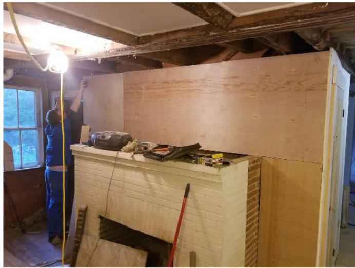
Luon installed prior to floorboards.
