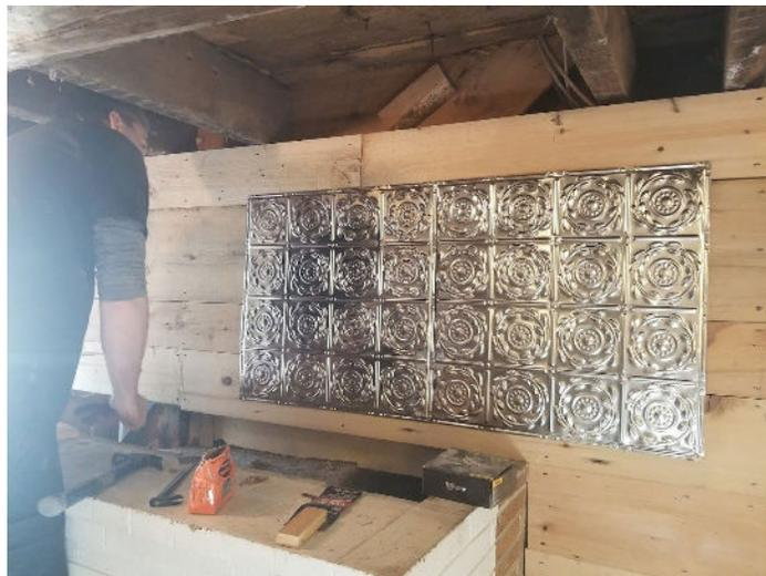
Once the wood was installed, we tested full panel tin sheets as a backsplash.
