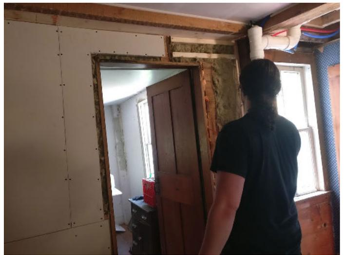
Pease inspecting the wall prior to installing another piece of drywall. This particular wall required substantial shimming before the drywall could be installed and inspired the crew to install the wood wall paneling by the fireplace.
