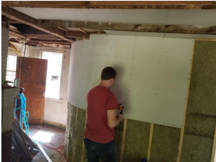
2018 installing the curved drywall.
