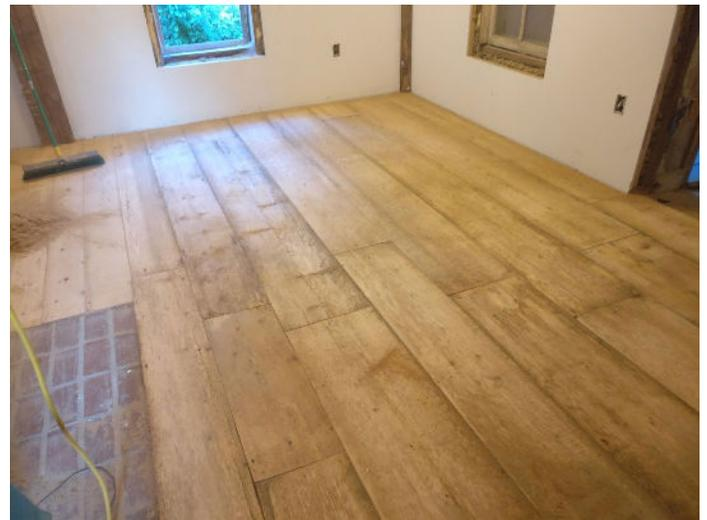
This photo shows the seamless transition between the 1" thick old growth pine and 3/4" thick wood donated by David Ferm. The transition piece was shimmed to eliminate any bump.
