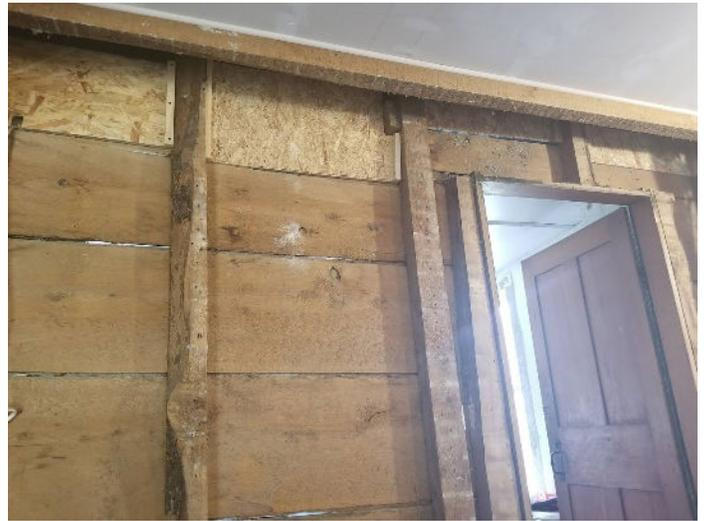
Additional plywood installed to close off the living room from the attic.
