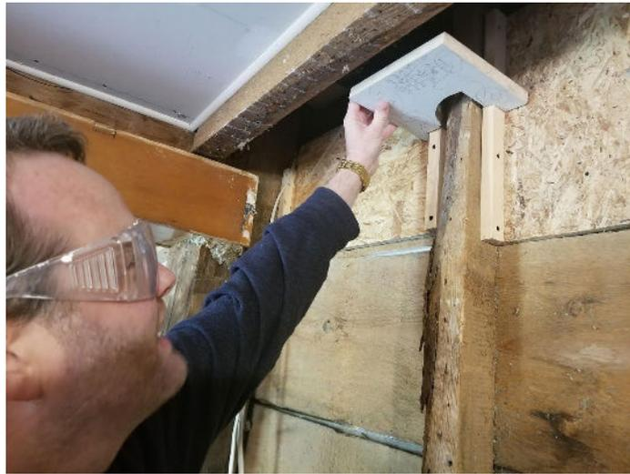
Walter demonstrates proper safety and the scribe piece used to make sure the fire-blocking would fit around existing studs.
