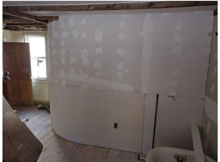
At the end of 2018, the curved wall looked almost done. Between the part you can't see on the left (the most extreme part of the curve), and the bucket of mud we spread over this thing, it about 100 more hours to get this thing finished.
