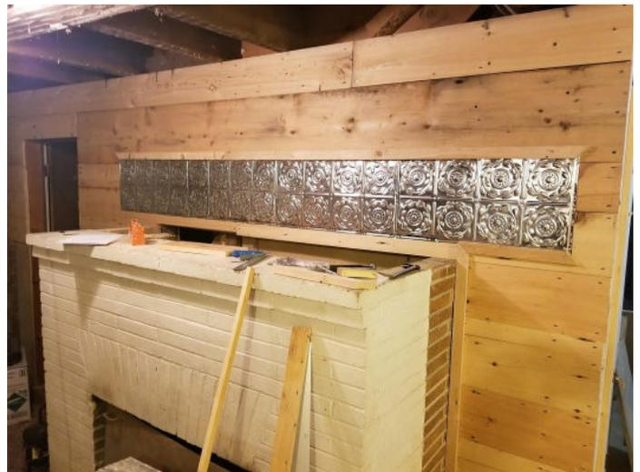
We ultimately cut the tin sheets in half and installed a trim border around the metal.
