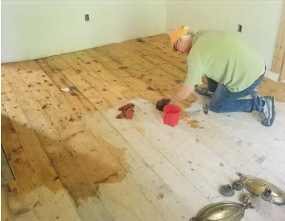
Board Treasurer Rod Pease works on cleaning the floors. They had gathered a thick layer of construction dust since being initially installed. We cleaned and sanded them before applying the natural oil.
