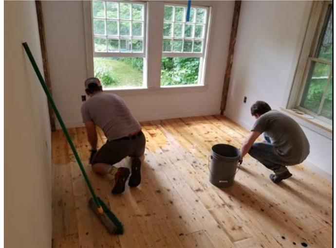
Applying the Tung Oil! We applied around eight coats, with 24-48 hours (if not more) in between coats
