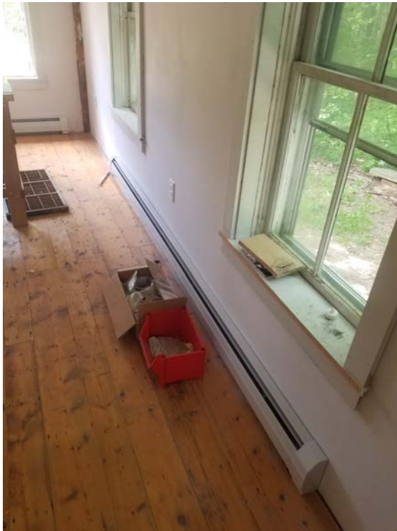
A stretch of new baseboard
