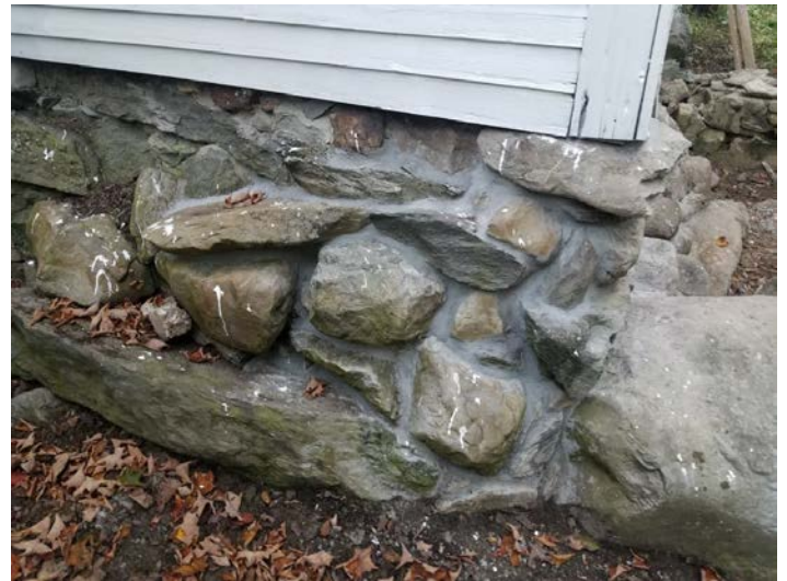
The remaining dry laid stone was re-grouted
