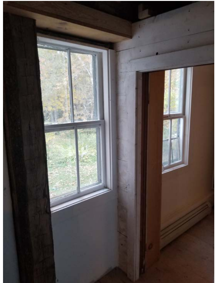
Windows scraped and repainted with lead sealing paint and trimmed out
