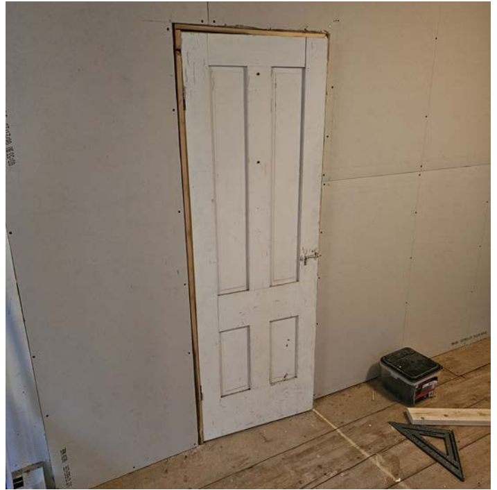
Temporary wall and door installed
