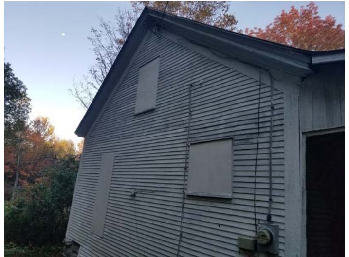
Busted windows boarded up, shed foundation removed, and house painted
