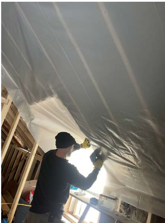
The ceilings and walls were insulated.
