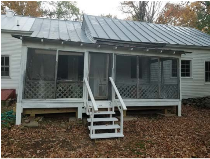
The back stairs were rebuilt with handrails added
