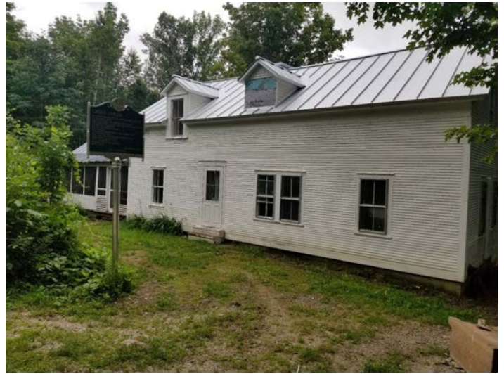
Newly installed roof and dormer roofs
