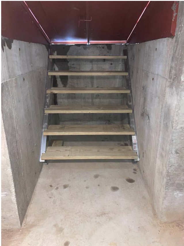
Stairs were installed in the hatchway.
