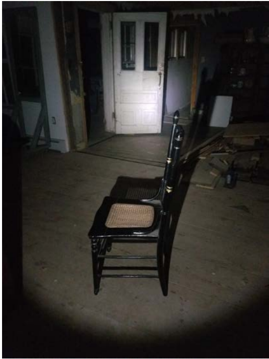
Opening access between living room and porch entrance
